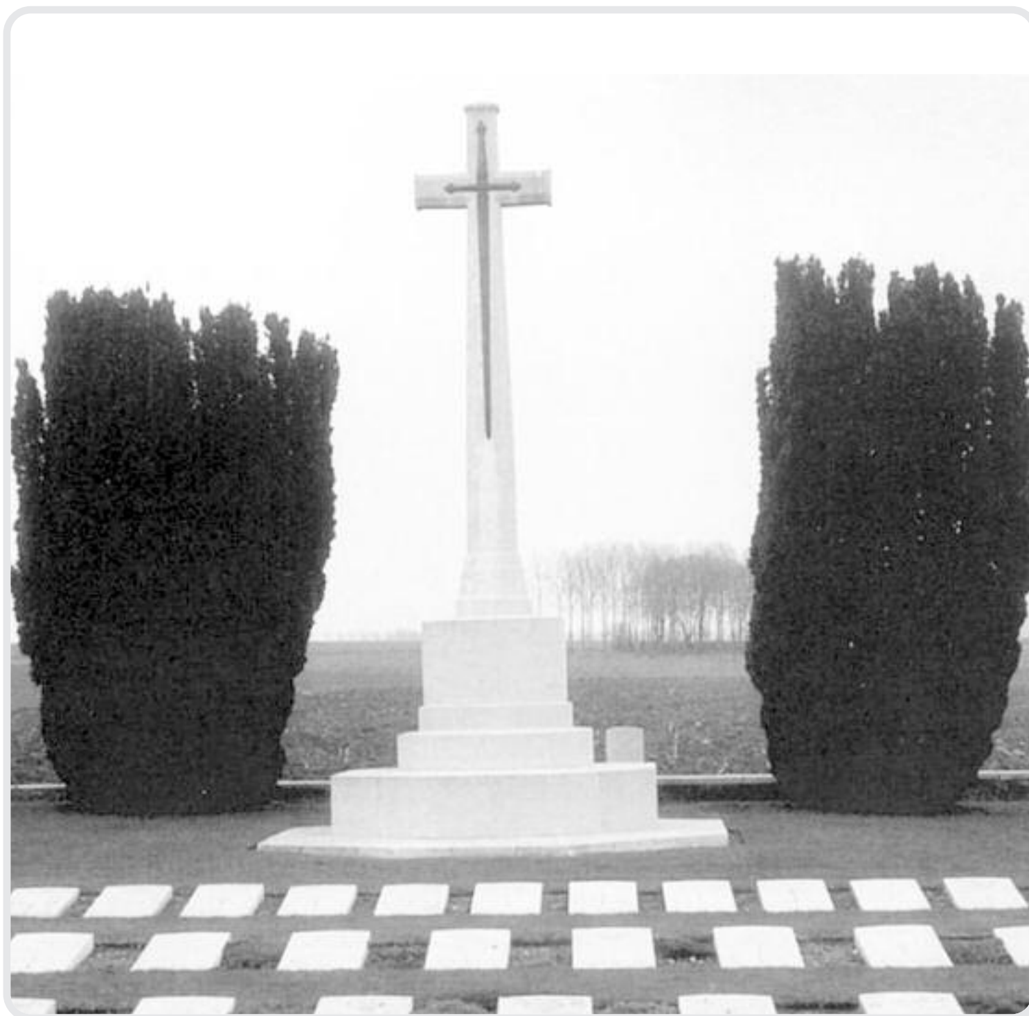
REMEMBERED: many of the headstones in Mill Road Cemetery have had to be laid flat due to subsidence caused by German tunnelling
